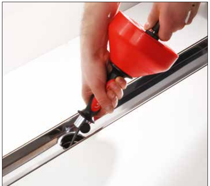
Clean the drain pipe with a small hand spiral
